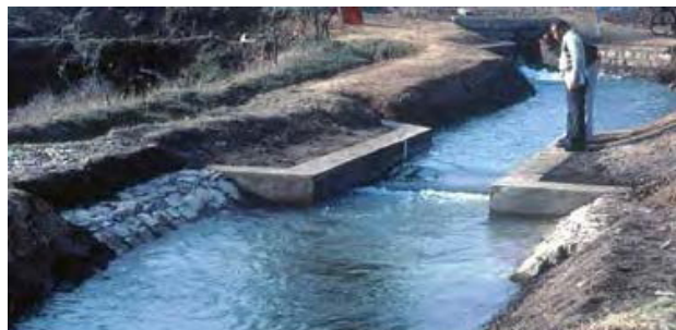
Figure 5. — A Rectangular-Throated Flume in India.
