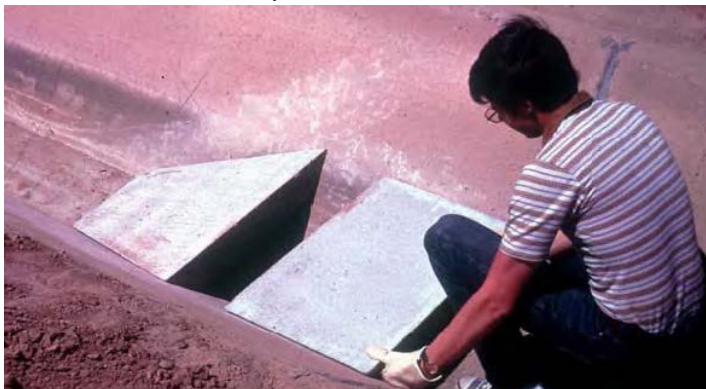
Figure 3. — Placing Pre-Cast Weir Sections in a Lined Trapezoidal Canal.
