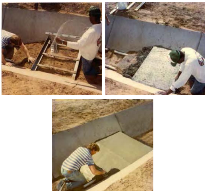
Figure 2. — Construction of a Broad-Crested Weir in a Concrete-Lined Trapezoidal Channel.
