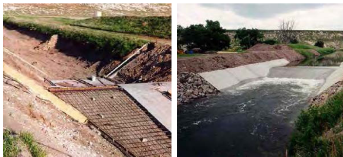
Figure 4. — Construction of a Large Broad-Crested Weir in an Earthen Channel.
