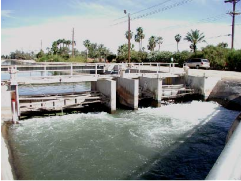
Figure 3. Multi-gate check structure 1-08 of the Salt River Project, Phoenix, AZ. Structures numbered from right to left.
