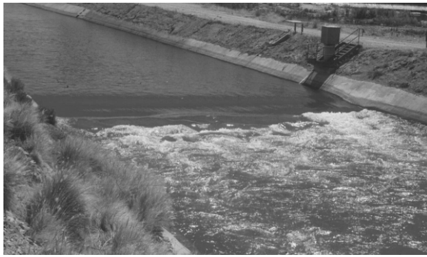
Figure 1. Flume in large canal. Note stilling well and the region of wavy water surface. Sill crest is located about midway between these two features. Canal flow depth is about 2.4 m (8 ft) and sill crest is about 1.4 m (4.5 ft) high.
