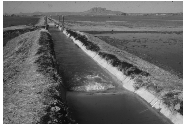
Figure 2. Flume in small concrete-lined canal.
